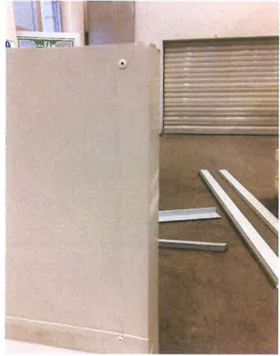
Photograph 2. Mounting of metal U profil on the bottom side of short wing.
